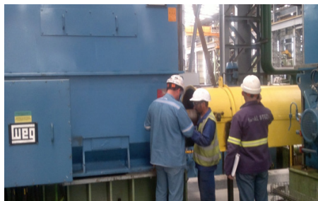
Onsite installation of Earthings at SAFFEL STEEL
