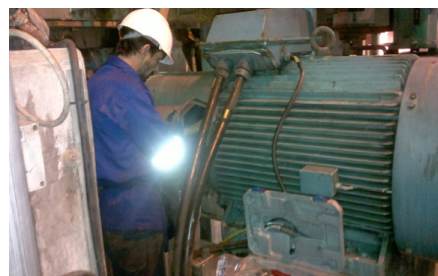
Onsite installation of Earthings at SAPPI SAICCOR
